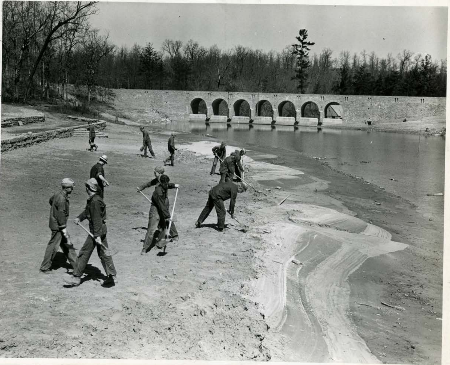
Civilian Conservation Corps (CCC) boys spreading sand on the beach at the Cumberland Homesteads State Park
